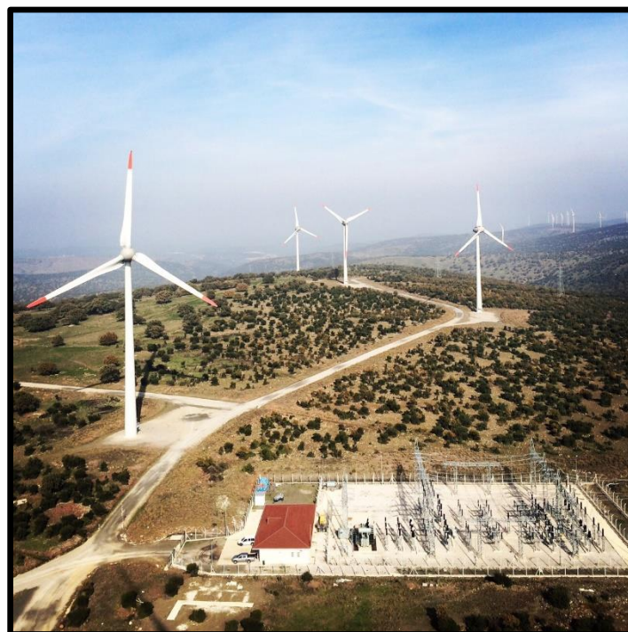
Figure 1. Example photos of wind turbines and switchyard
